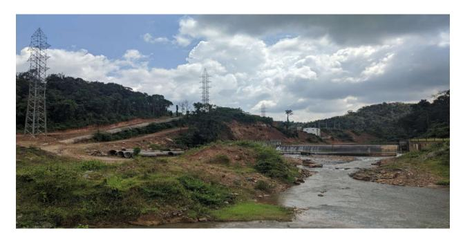
Pipelines and power lines being installed at Keriholla weir. The pipelines will pump the water up the Western Ghats hills before flowing in the open channels in the plains. Photo by Mohit M. Rao/Mongabay
