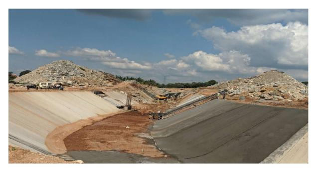
A 150-m width of land will be required to carve out a 30-m wide channel that is designed to carry 24.01TMC of water from the Western Ghats. Construction of the channel is ongoing near Arsikere in Hassan district. Due to farmer's protest, construction has stalled at the Tumakuru border a few kilometres away. Photo by Mohit M. Rao/Mongabay
